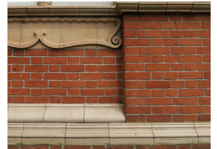
Venue 28 Brickwork Detail - Brick + Terracotta
